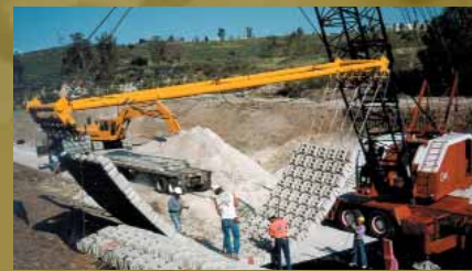
INSTALLING & LIFTING DEVICE
